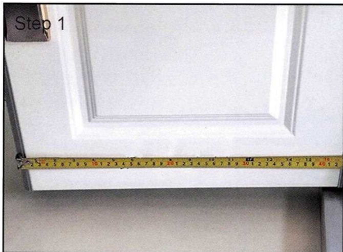
Step 1 Cut the length according to the door width, suggest to cut about 2mm shorter than the door width.
